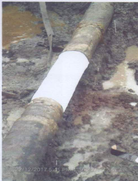
SPILL POINT AFTER REPAIRS: fig3
