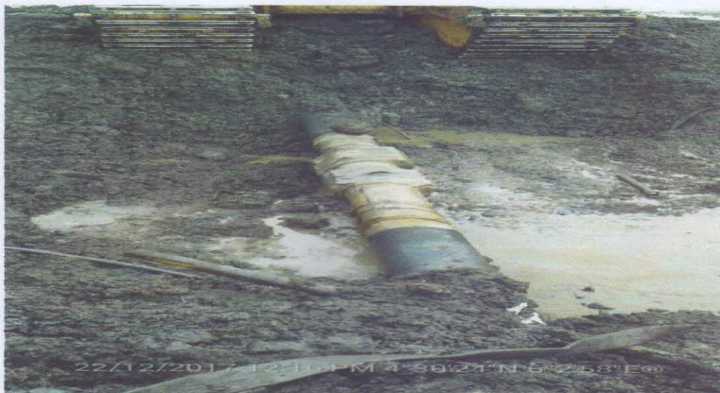
SPILL POINT AFTER EXCAVATION: fig1
